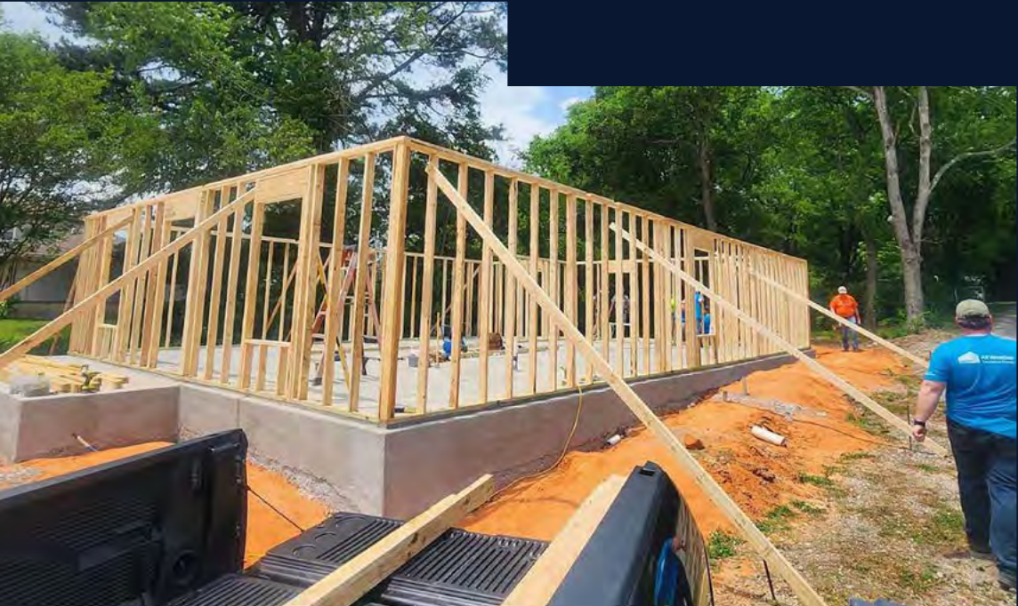
Our All Weather Insulated Panels (AWIP) business in the US provided labour and materials to the non-profit housing organisation, Habitat for Humanity
