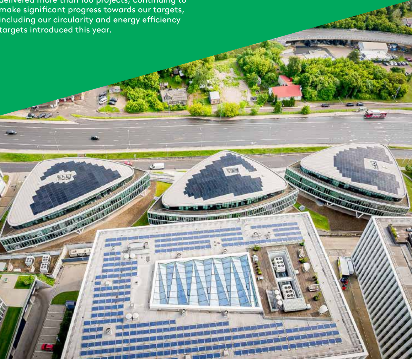
BALTIC HEARTS OFFICES Vilnius, Lithuania Insulated Building Envelopes Dome Solar roof-solar PVC
