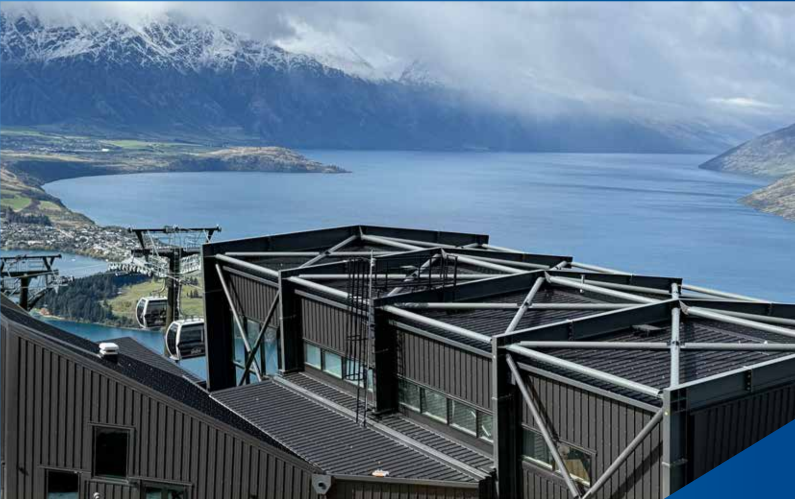
SKYLINE GONDOLA Queenstown, New Zealand Insulated Building Envelopes KS1000RW Trapezoidal Roof Panel Photography: Wyatt + Gray Architects
